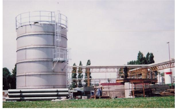
Tank in AISI 316L to 300 m<sup>3</sup>
